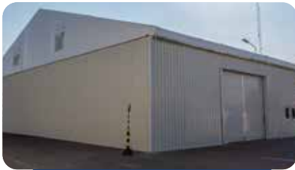
Temporary Warehouse Alluminum Frame
