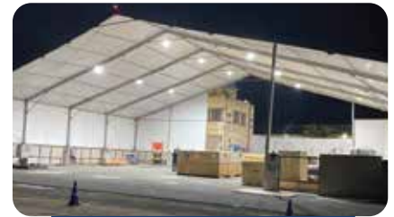
Aircraft Maintenance Hangar
